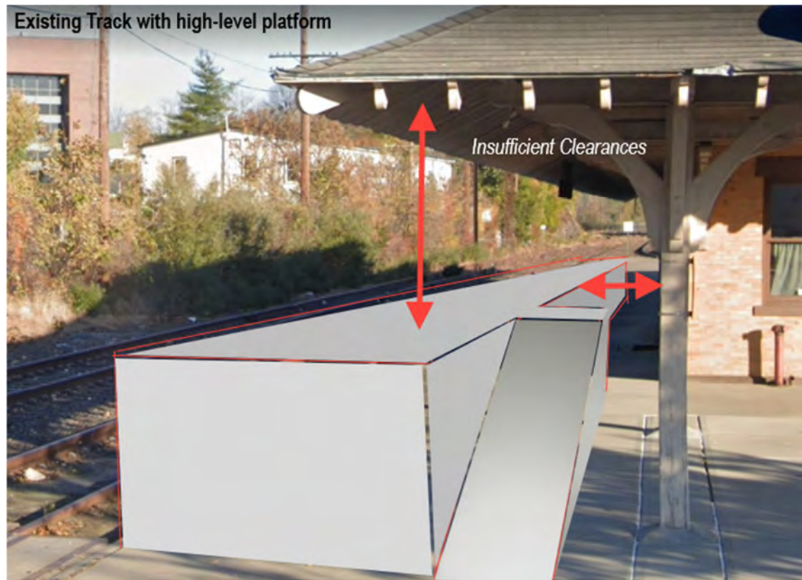
FIGURE 41. DANBURY RAILWAY MUSEUM TRACK WITH HIGH-LEVEL PLATFORM
