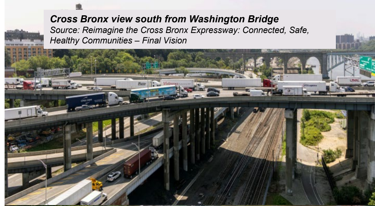
Macombs Avenue over the Cross Bronx Expressway
