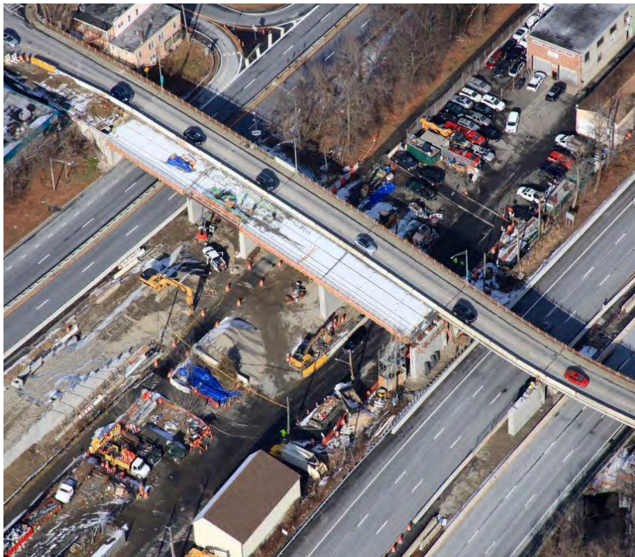
Ashford Avenue Bridge over the Saw Mill River Parkway
