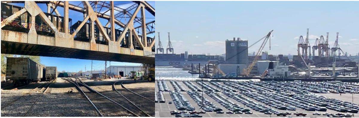
Figure 3 Fresh Pond Yard in Queens (Left) and Port Newark/Elizabeth (Right), Examples of Freight-Handling Land Uses
