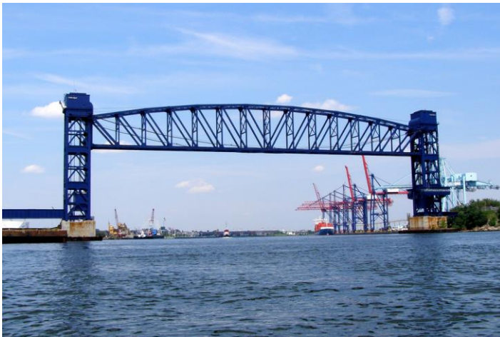
Arthur Kill Lift Bridge, Staten Island
