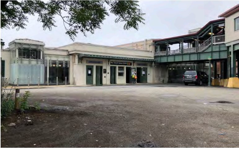
Existing New Utrecht Avenue Station
