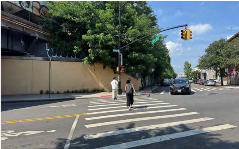
Site of future Myrtle Avenue Station
