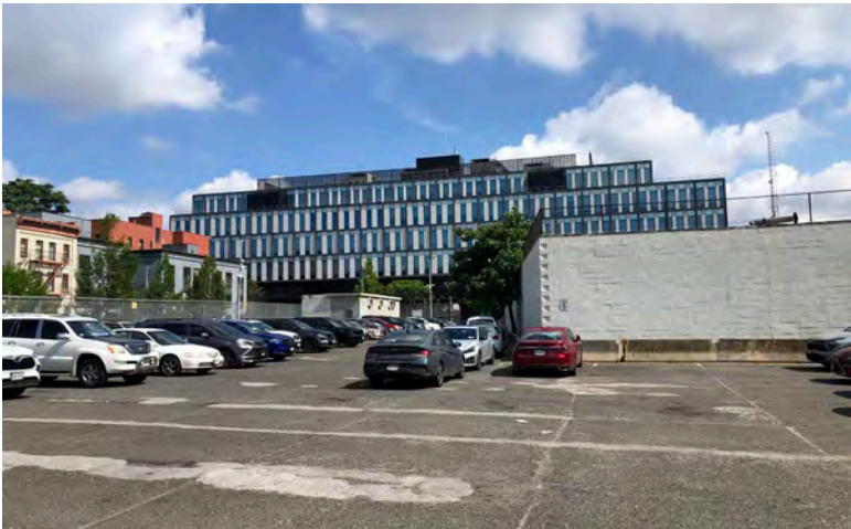
Site of future Atlantic Avenue Station
