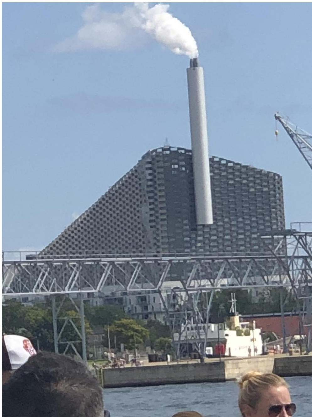
A Manhattan SWAB Member took this photo of CopenHill in the summer of 2025, during a visit to Copenhagen, Denmark. The photo shows that the plant is emitting a continuous stream of "smoke" on a day when the temperature was in the 70's F.
