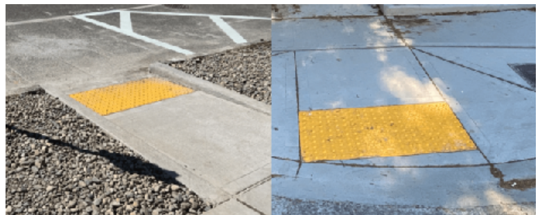
Figure 12: Examples of 'Tactile Walking Surface Indicators' or ADA warning pads—source: Seattle Department of Transportation.
