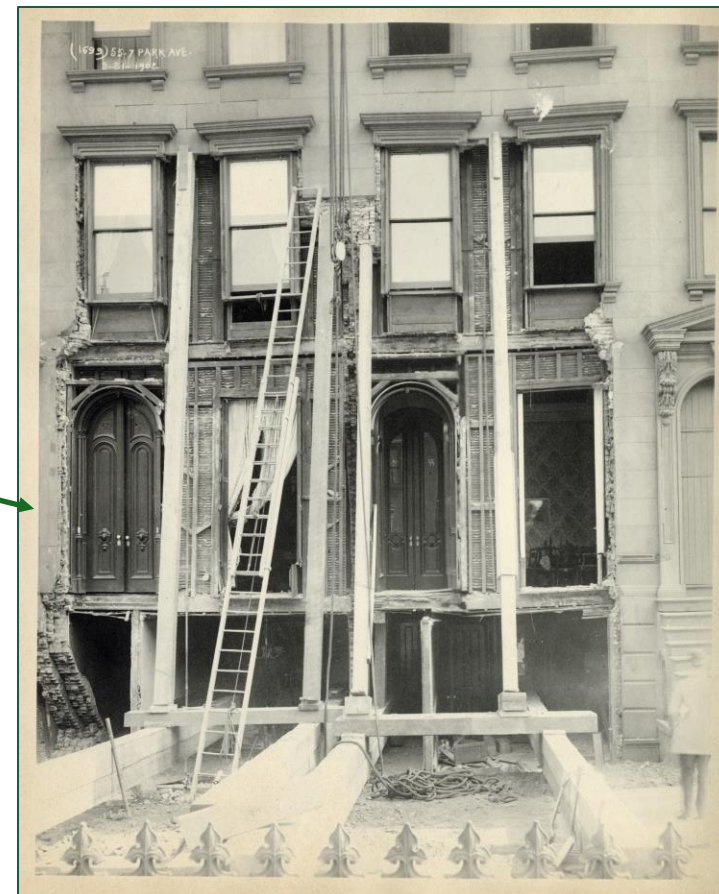
[#55-7 Park Ave.], 3/21/1902, R1S3_1699, Subway Construction Photograph Collection, New York Transit Museum
