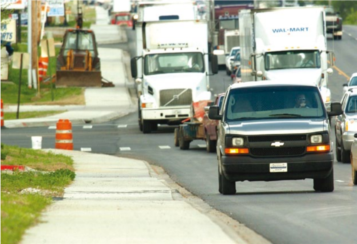
This is a typical example of a high-speed, high-traffic arterial road. Though it does contain a sidewalk, it's a narrow sidewalk with frequent curb cuts for turning cars and little room for error.
