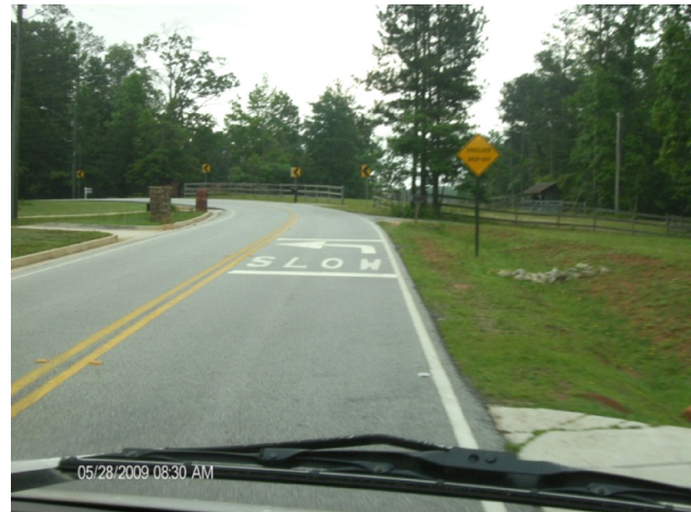
Figure 4: Curve Ahead Pavement Markings and Signage
