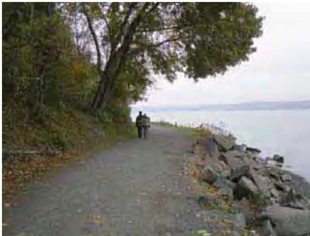
Stabilized stone screening as seen in Nyack State Park
