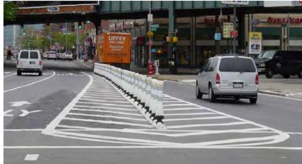
Figure 5.14 Use of Flexible Bollards and Paint for Cost Effective Changes
