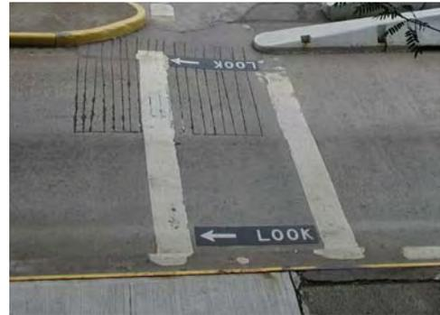
Figure 5.19 In-Pavement Warning
