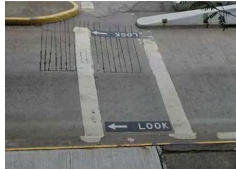
Figure 5.19 In-Pavement Warning
