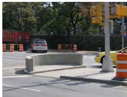
Figure 5.4 Raised Median with Non-raised Path for Wheelchairs
