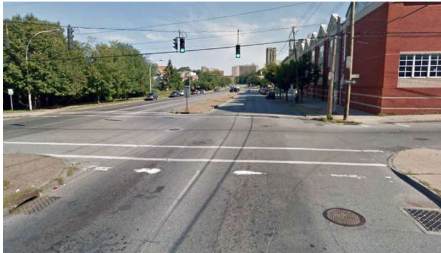
Riverdale Avenue at Morris Street Facing North
