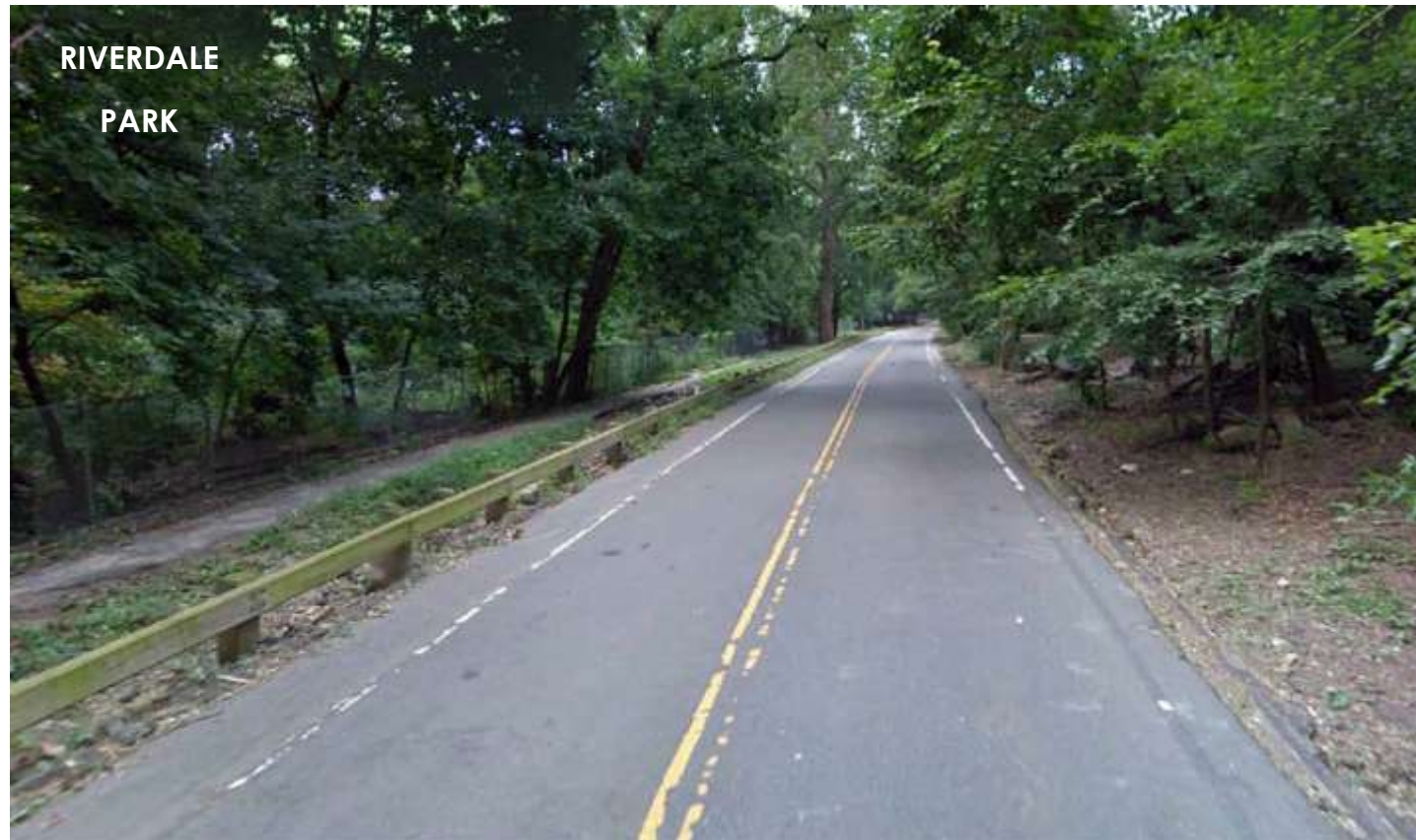
View looking north on Palisade Avenue Between Spaulding Lane & 232 nd Street
