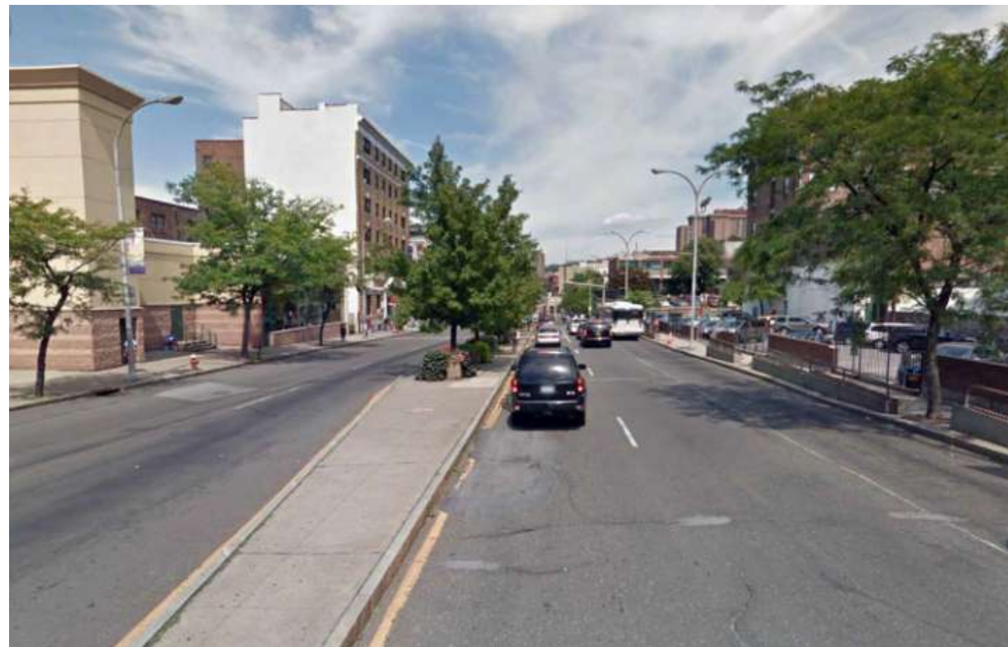
Riverdale Avenue North of Prospect Street Facing North
