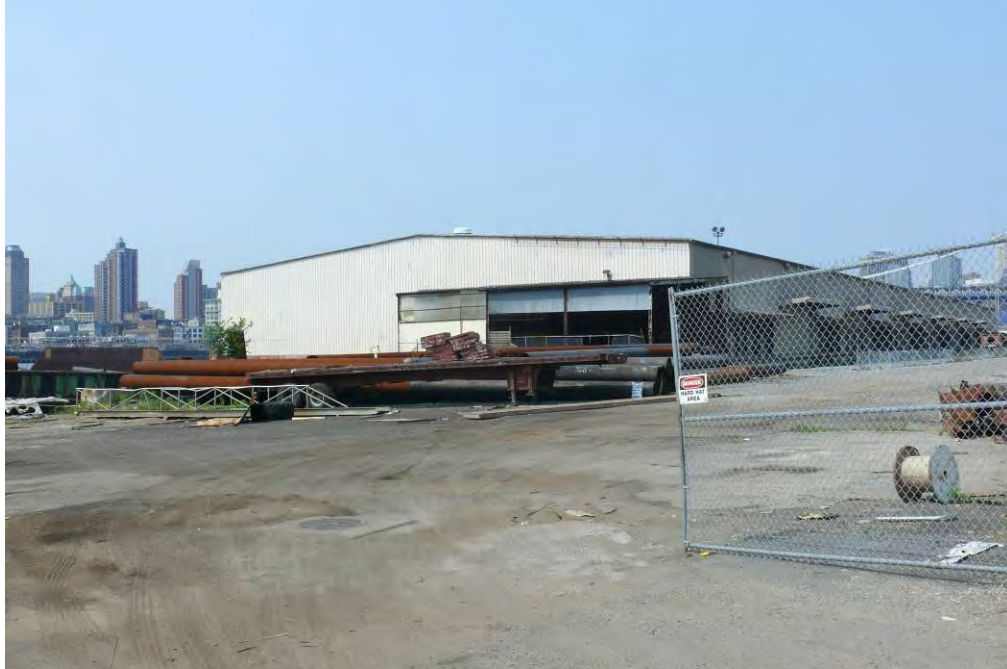
Figure 8. Location 3 Pier 43 (Old Fruit Pier) at Montgomery Street
