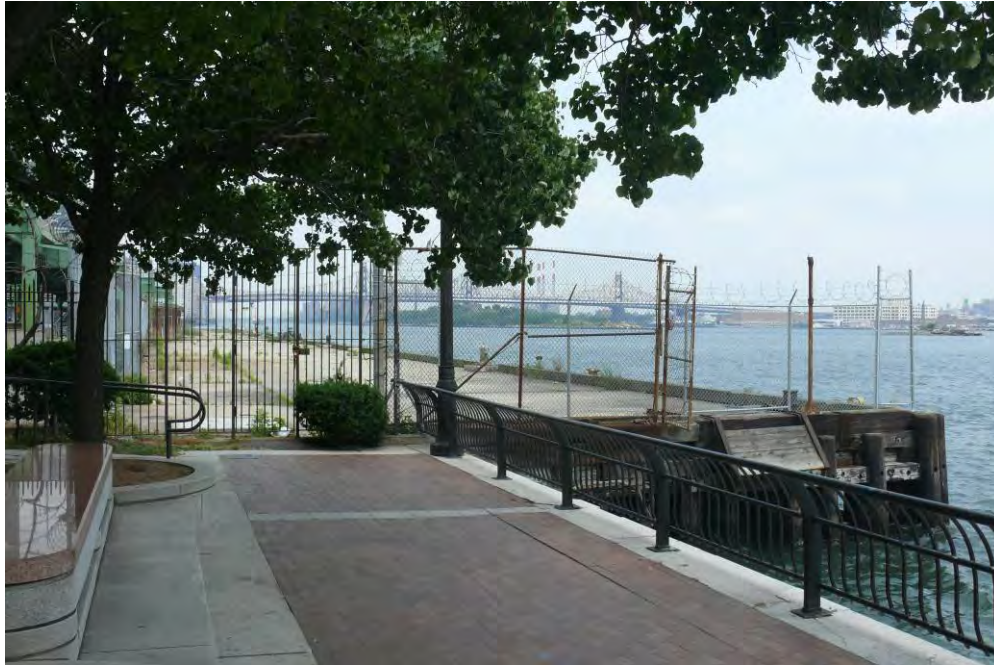
Figure 7. Location 1 Unused Pier at 37 th Street
