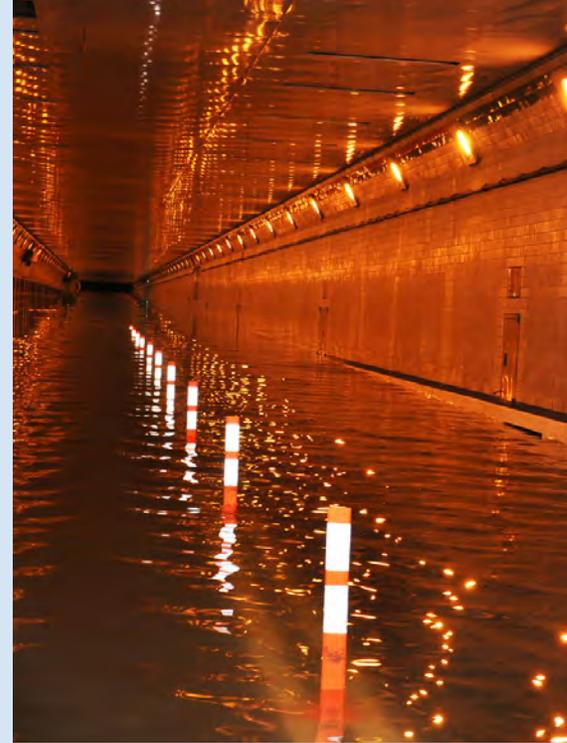
Among the region's vehicular crossings, the Hugh L. Carey Tunnel, Queens Midtown Tunnel and Holland Tunnel flooded with seawater. The city's coastal and circumferential arterial roadways were washed over. Roadways and bridges sustained damage after being over-topped by floodwaters or being struck by breakaway barges and other transported debris. Numerous overhead sign structures were damaged. Bridges and tunnels around the city were closed because of the danger from high winds and flooding.
