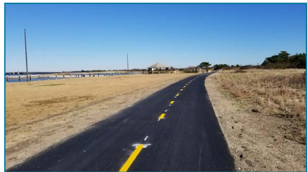
Jones Beach Shared-Use Path at the West End of Jones Beach
