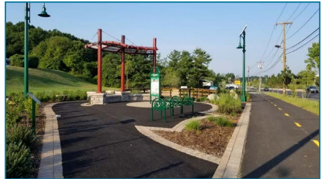
Green Stop in Nesconset on the NY 347 Parks to Port Greenway
