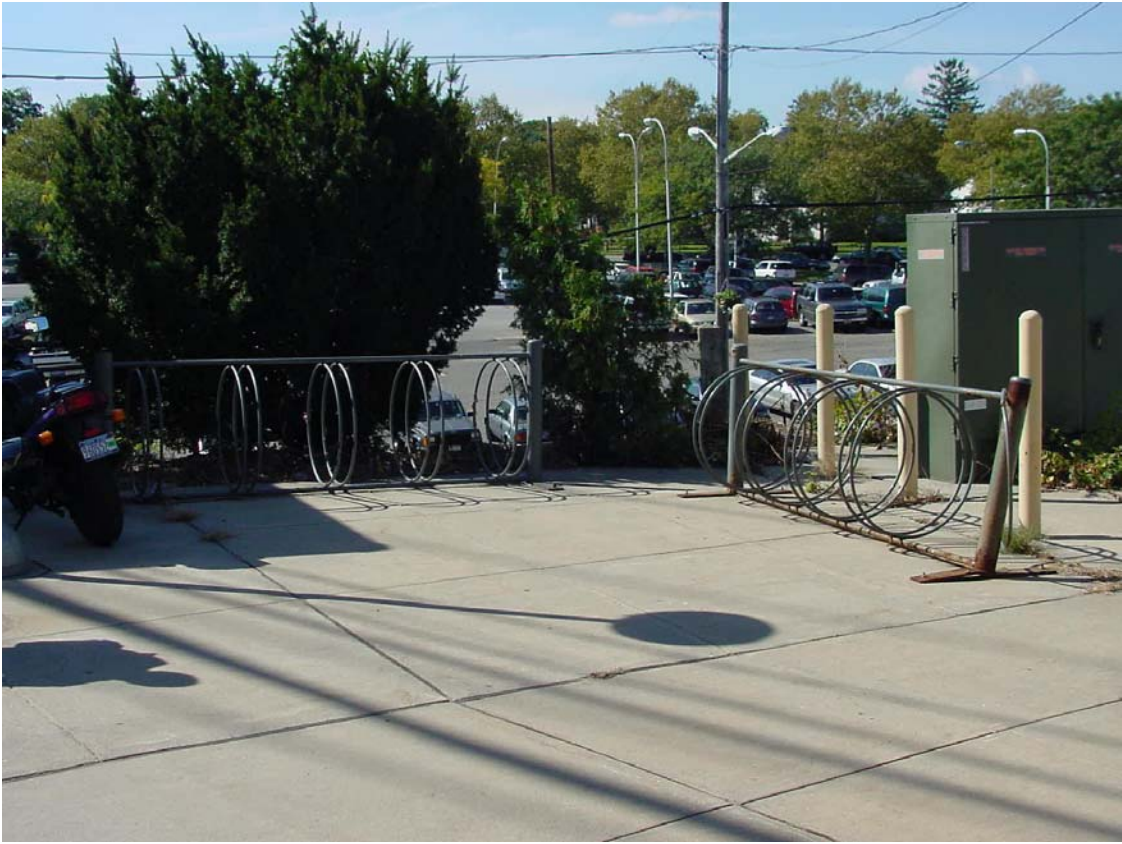
Figure 5. Huntington Station Bicycle Racks.
